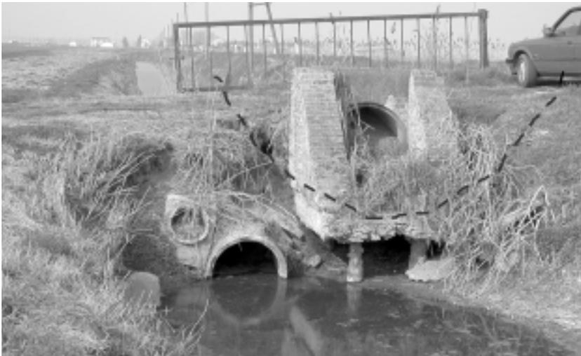
Fig. 5 – The effect of land subsidence in the Zennare Basin: an old masonry culvert presently above the water level and substituted by two lower concrete drainpipes, the higher of which already unusable. A qualitative position of the ditch section in the original configuration is sketched.
