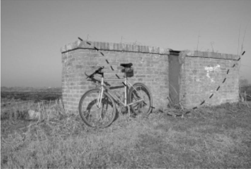
Fig. 4 – Effects of land subsidence in the Zennare Basin: an old abandoned weir originally constructed to close a drainage ditch completely protruded above the ground level. A qualitative position of the ditch section in the original configuration is sketched.
